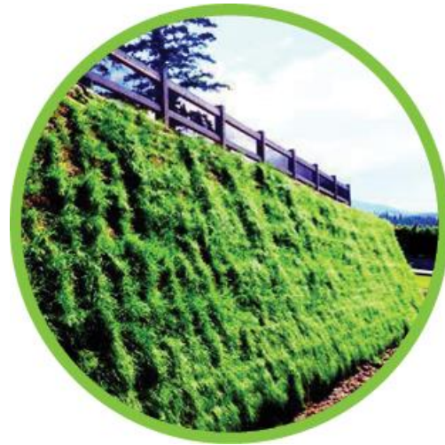
Vegetated Retaining Wall
